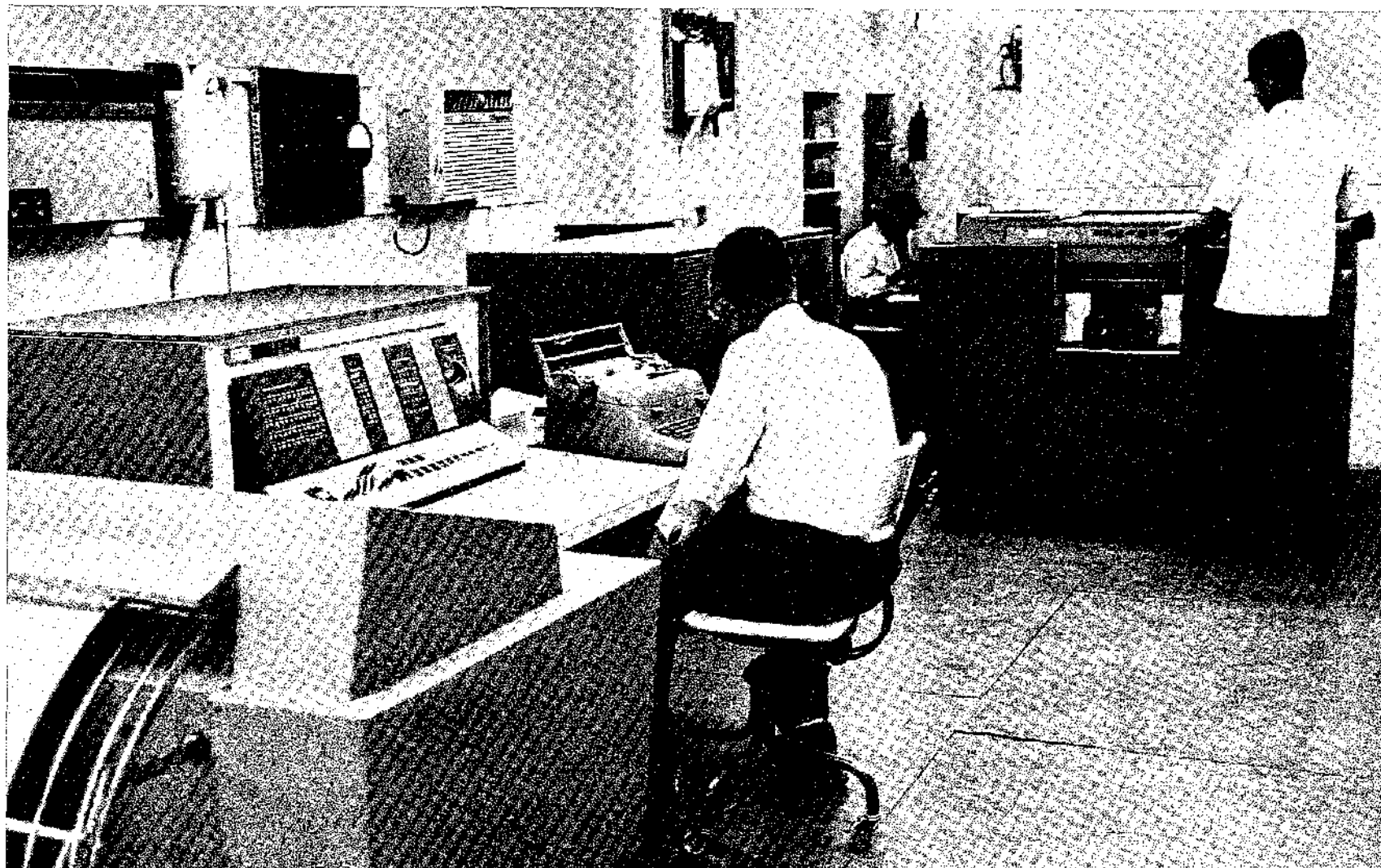
The Computer Room at the Institute of Tropical Meteorology in Poona, India, which was established under a UNDP/WMO Special Fund Project completed in 1967.
